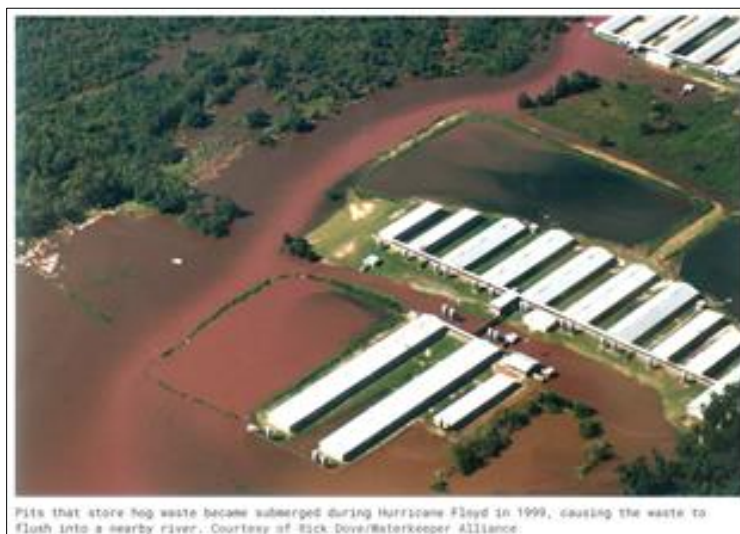
Figure 2 Flood damage to manure farms, displaying massive hog waste runoff
