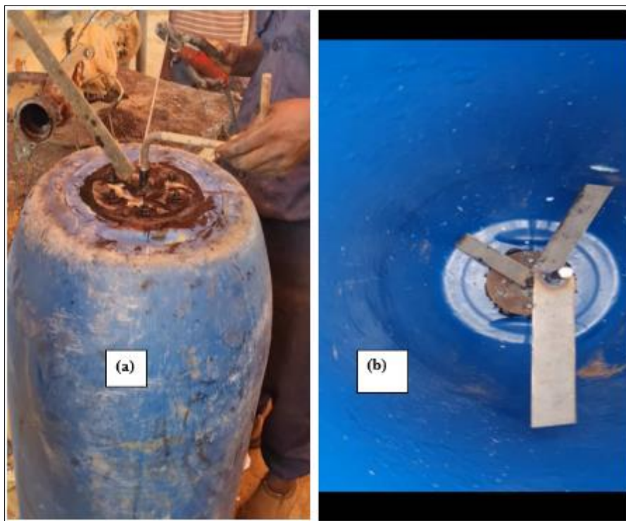
Figure 6 Installation of Stirrer to Digester (a: outside view; b: inside view)
